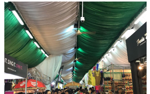
Combination of LED flood lights and linear LED tube light that becomes a Hero for picking up fabric texture.
