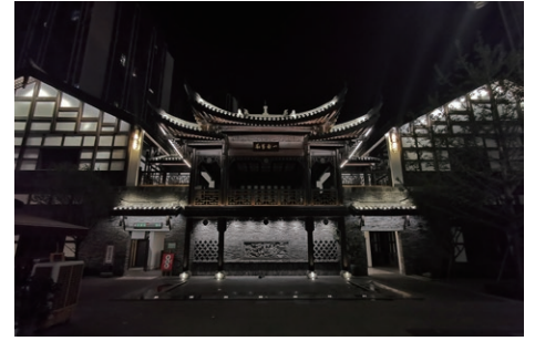
Linear architectural lights outlines the details of chinese construction
