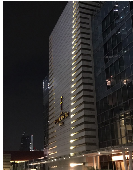
Facade light creates direct glare when we see from the side.
