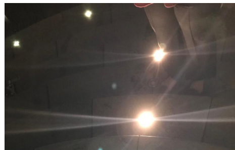
Inground light embedded in to the steps create glare.
