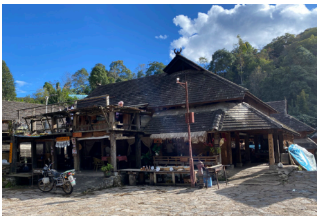
Private house with teahouse on the first floor and a living space on the second floor
