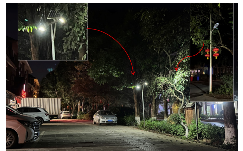
Different kinds of fixtures on the sidewalks
